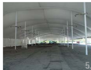
1. Dramatically shaped high peak design 2. Both twin pole and single pole designs are available 3. Clean and simple aluminum perimeter plates make connections to guyouts easy 4. Typical stake bar and web winch used for anchoring the tent system 5. Interior of 100' wide twin pole design 6. Heavy duty centerpoles and specially designed pole pins.
